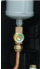
An inspection glass for the refrigerant is located behind the front cover on the copper tube under the drying filter. When the collector is working constantly, the liquid in the inspection glass will be transparent; there should be no bubbles or foam. When the compressor starts and before the pressure has stabilized, bubbles and foam can be seen.
