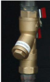
In order to protect the condenser there is a pollution filter in the return circuit. It's located behind the front panel under the pump for the heating circuit. If the warning lamp for the high-pressure alarm lights, it could be that the filter is clogged. This sometimes occurs shortly after the installation of the heat pump if there is dirt in the old circuits.
